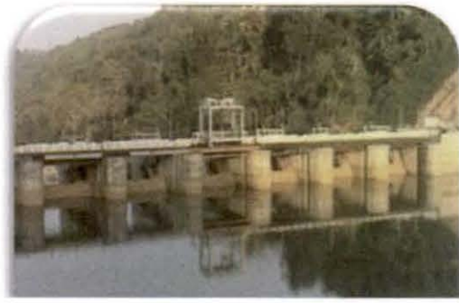
Water reservoir in Karbi Langpi Project
