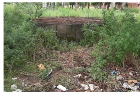
Artificial recharge structure at Amloh canal rest house, Patiala
