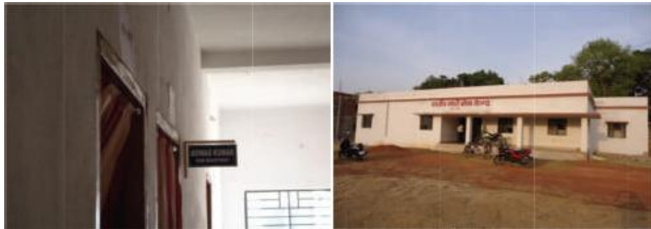
Photographs showing BNRGSK building running as Office of the Sub Registrar, Urban Area, Kanke, Ranchi
