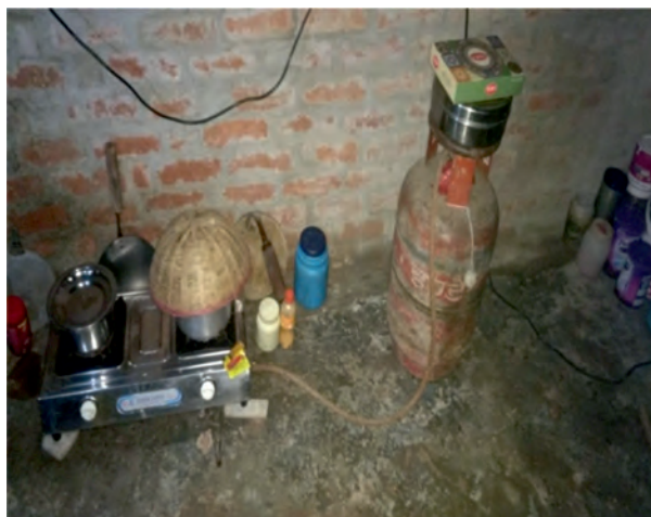
1. Gas stove Kept on floor: IOCL, Kanpur
