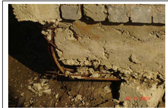
Picture showing eccentricity of Column at Mathpurena site – BSUP Raipur (The compressive strength of concrete work was found 111.15 kg/sqcm against the standard of 200 kg/sqcm.
