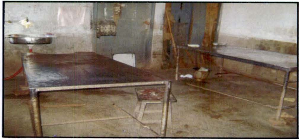
Labour room of RH, Sahpur, Bhojpur
