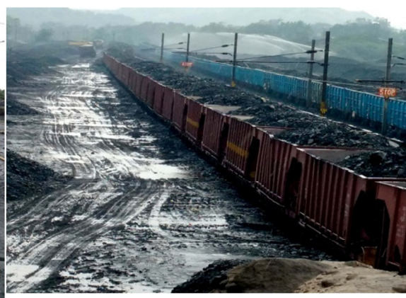
Pic. 04: Ghugus Railway siding of WCL with fixed sprinklers
