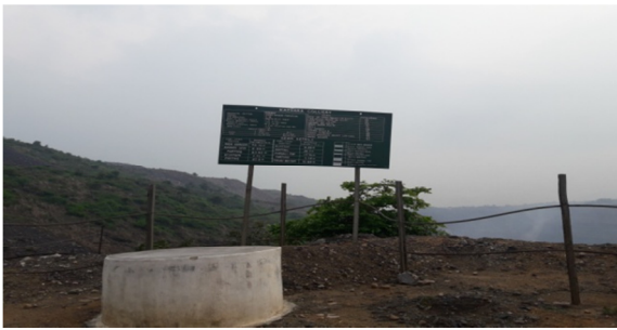
Pic. 11: Para No. 6.3.2, Table No. 14, Sl. No. 01: OB dumps without Plantation at Kathara OCP of CCL
