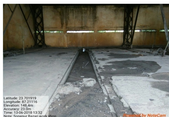
Pic. 07: Para No. 5.5.1 (Sl. No. 02): Choked drains and chambers of HEMM washing facility at Sonapur Bazari, ECL, resulting in overflow of sludge
