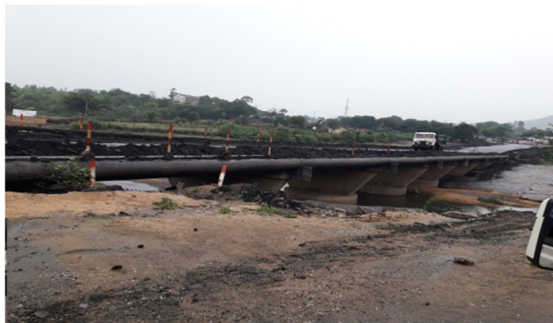
Pic. 08: Para No. 5.7.1: Spillage from overloaded trucks coal accumulated along the sides of the bridge of Safi River at Piparwar OCM of CCL
