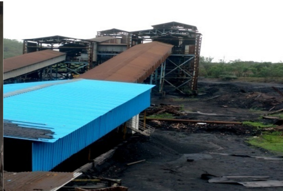
Pic. 02: Covered conveyor belt at CHP in Mungoli mine of WCL
