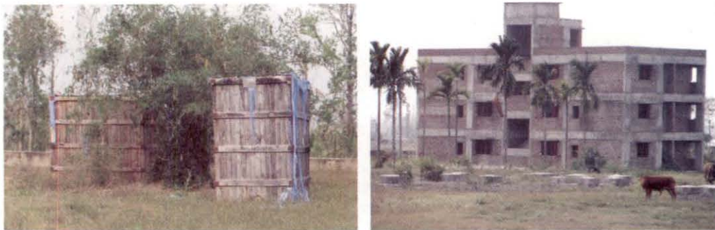
Idle machinery, equipment (two alternator machines) and building (Type III residential three storied block) of the abandoned project “22.92 MW HFO based thermal Power Plant at Dimapur” (June 2008).
