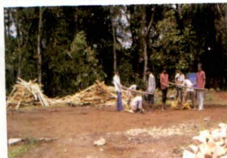
Work in progress -Jowai Water supply scheme, Meghalaya
