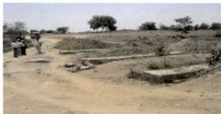
Photograph of incomplete bridge in Amarda village road
