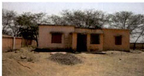
Ambajhari sub-centre located outskirts
