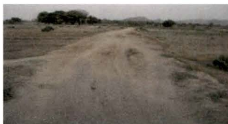
(Improvement of road from Balandapada road in Gochhapada Gram Panchayat)
