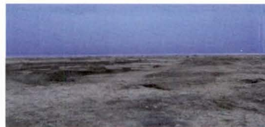
Excavation of new tank at Khambeswarpali, Kantamal Block
