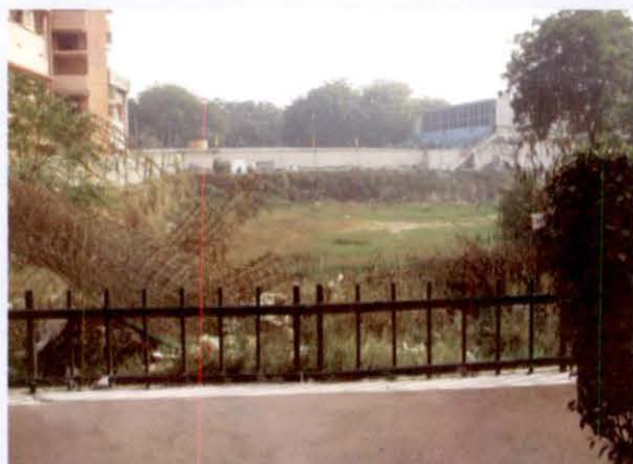
A view of excavations which endangered school property and lives of the students
