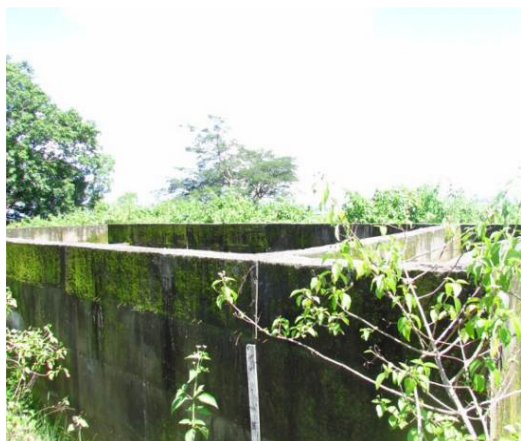
Incomplete settling tank
