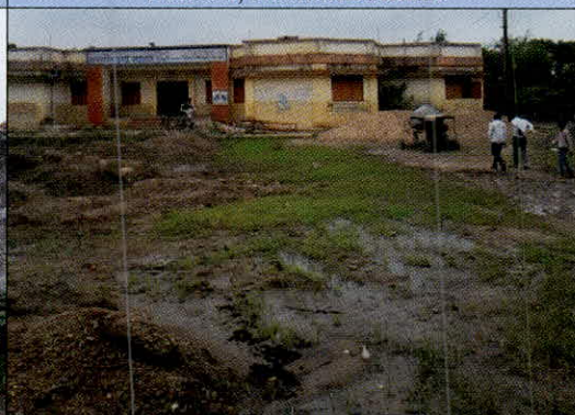
School building of High School Jamunia Kalan in which the classes of Middle school shifted
