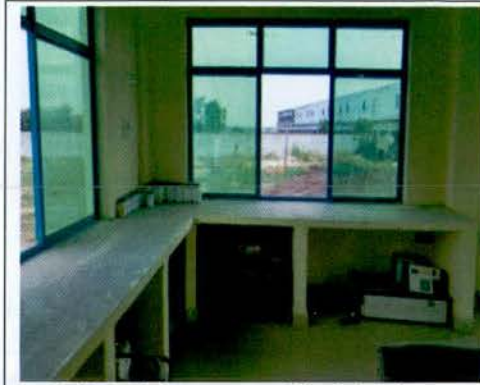
Defunct laboratory at Shivri, Lucknow
