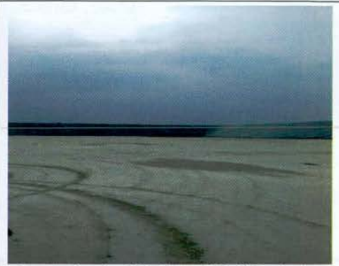
Incomplete landfill site at Shivri, Lucknow
