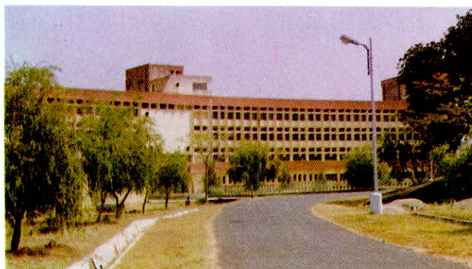
A view of the unoccupied building constructed at a cost of Rs 348.45 lakh lying idle since March 1996
