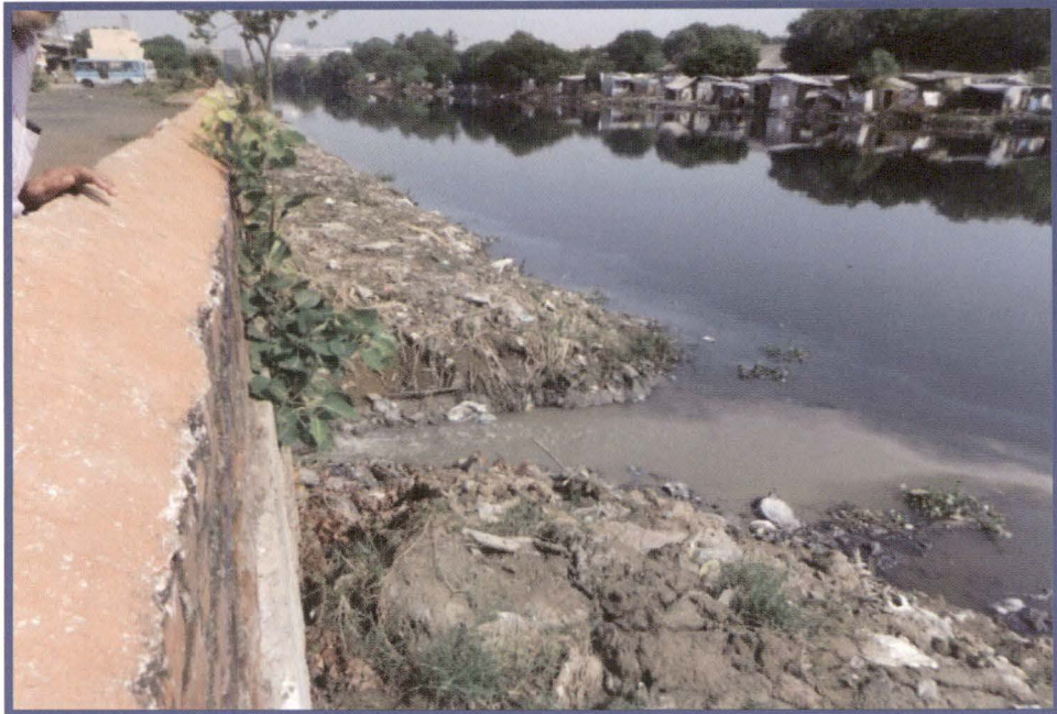
Encroachment and sewage outfall (Pallavan Nagar)
