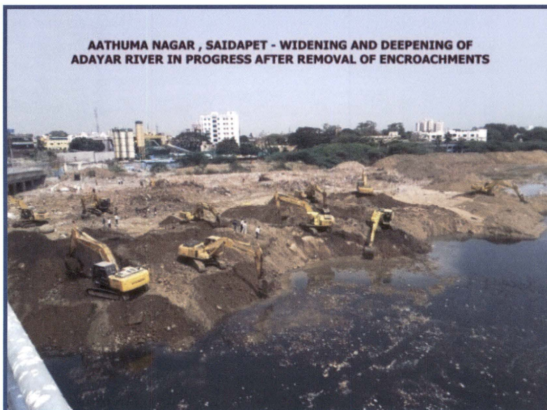
Exhibit 8.1 - Post flood works in Adyar River
