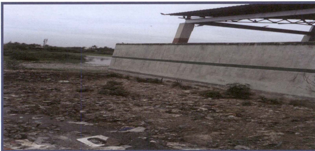
Exhibit 4.5: SWM facility inside Peerkankaranai Lake
