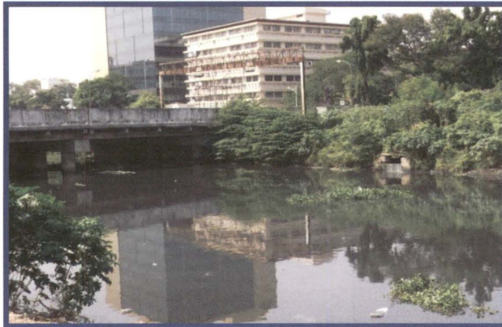
Blocked vent and sewage outfall (Langs Garden)
