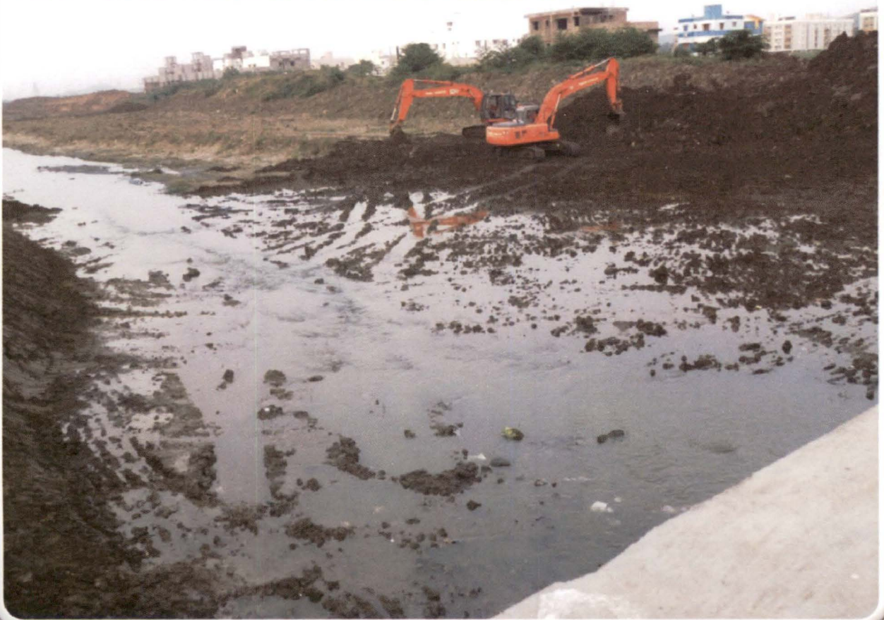
Post - flood works at Nandambakkam canal
