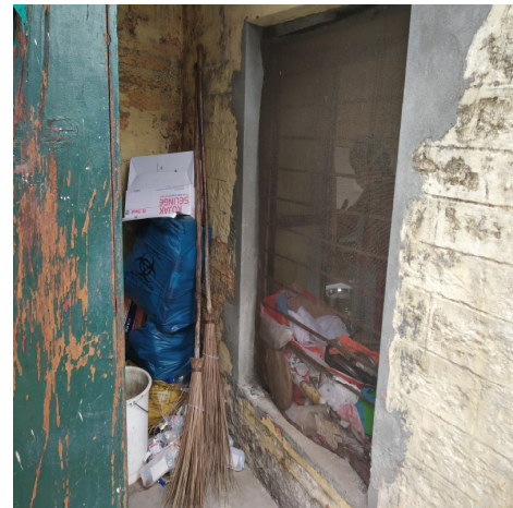
Photograph-2: District Female Hospital, Almora
