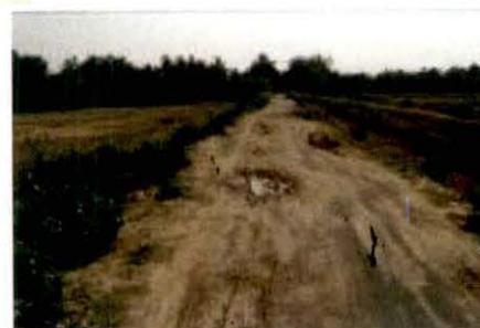
ICI canal embankment road from Dhoda to Nandipur not providing all weather access after spending Rs 7.26 lakh by Dasarathpur block and overlapping execution by Irrigation Department
