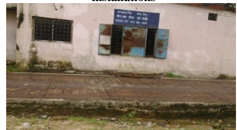
Abandoned mechanical weigh bridge
