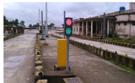
Damaged boom barrier in the back of defective signalling system
