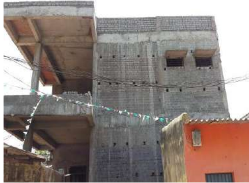
(Incomplete zone office building at Raigarh town)
