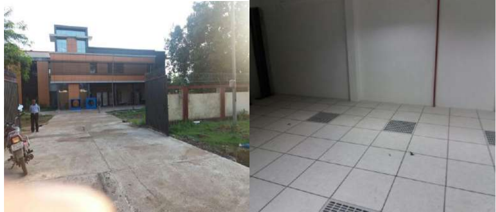
(SCADA Control Centre Building Bhilai without SCADA installations)
