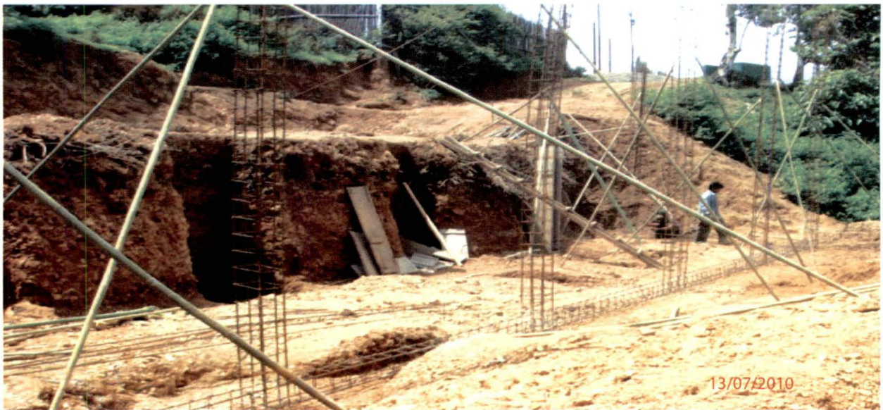
Constn. of Higher Secondary School hostel at Ngopa
