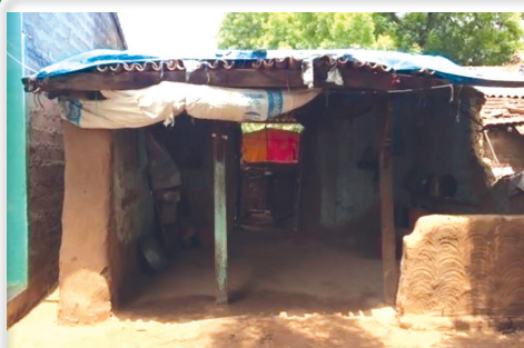
Picture 3: Kutcha house of a beneficiary in Malgadh village, Deesa taluka under Banaskantha district on the date of joint visit (06 July 2017). The beneficiary had submitted fake photograph of the completed house (Picture 4) to claim third instalment.
