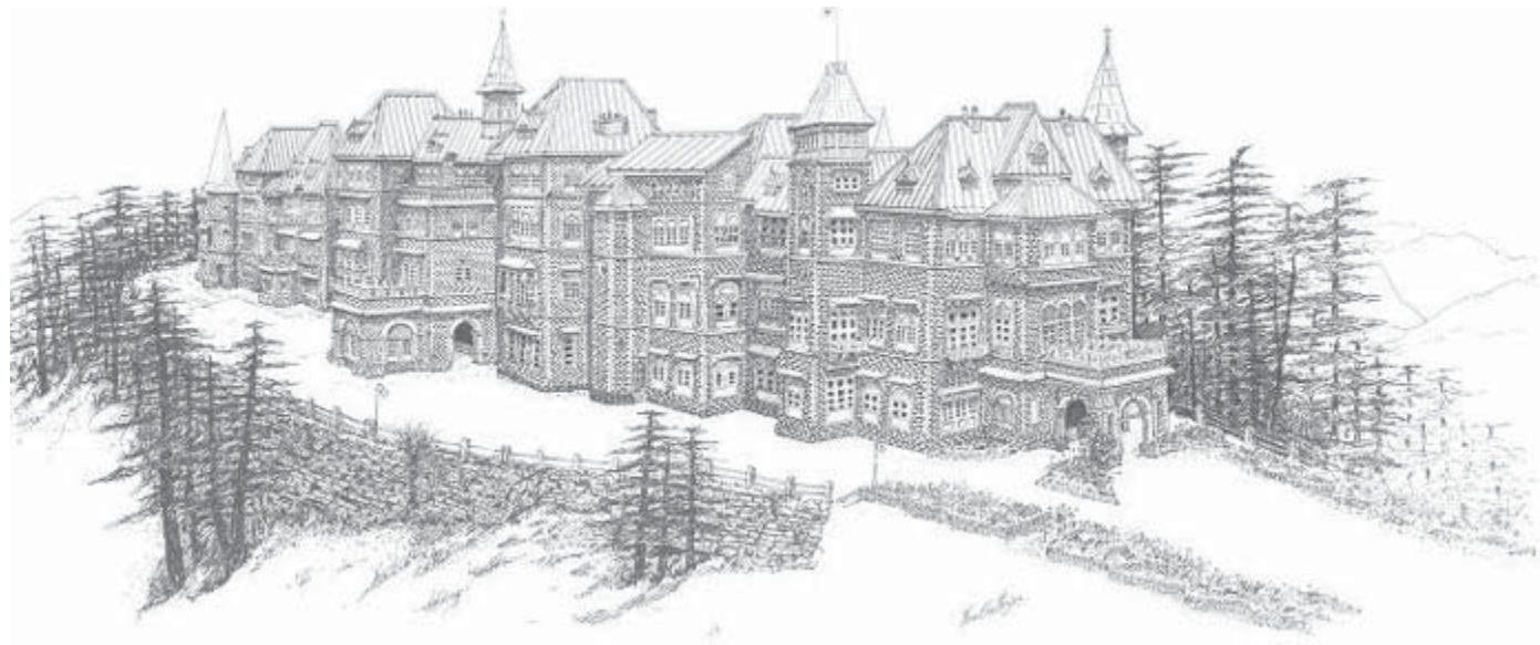
An artist's sketch of Gorton Castle Building Shimla which houses the office of Accountant General Himachal Pradesh. It housed the Central Secretariat of the British government during summer upto 1942; subsequently, it was the Headquarters of Auditor General of India for sometime.
